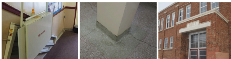
Existing Spruce Avenue 7–9 School Site
